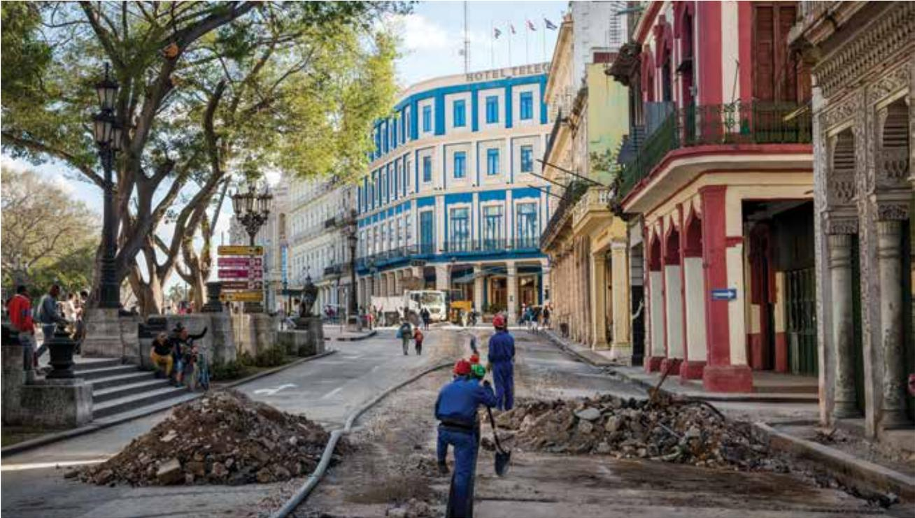
Cuban workers bury new utility lines in a trench cut in the pavement of Paseo Martí in this view looking southward along the Paseo del Prado in Havana in 2016. In the background is the Hotel Telégrafo, which reopened in 2002 after a total restoration.
